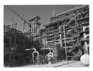
Construction is nearly complete on the 7.8-million-tons-per-year RasGas liquefied natural gas (LNG) Trains 6 and 7 in Qatar.
