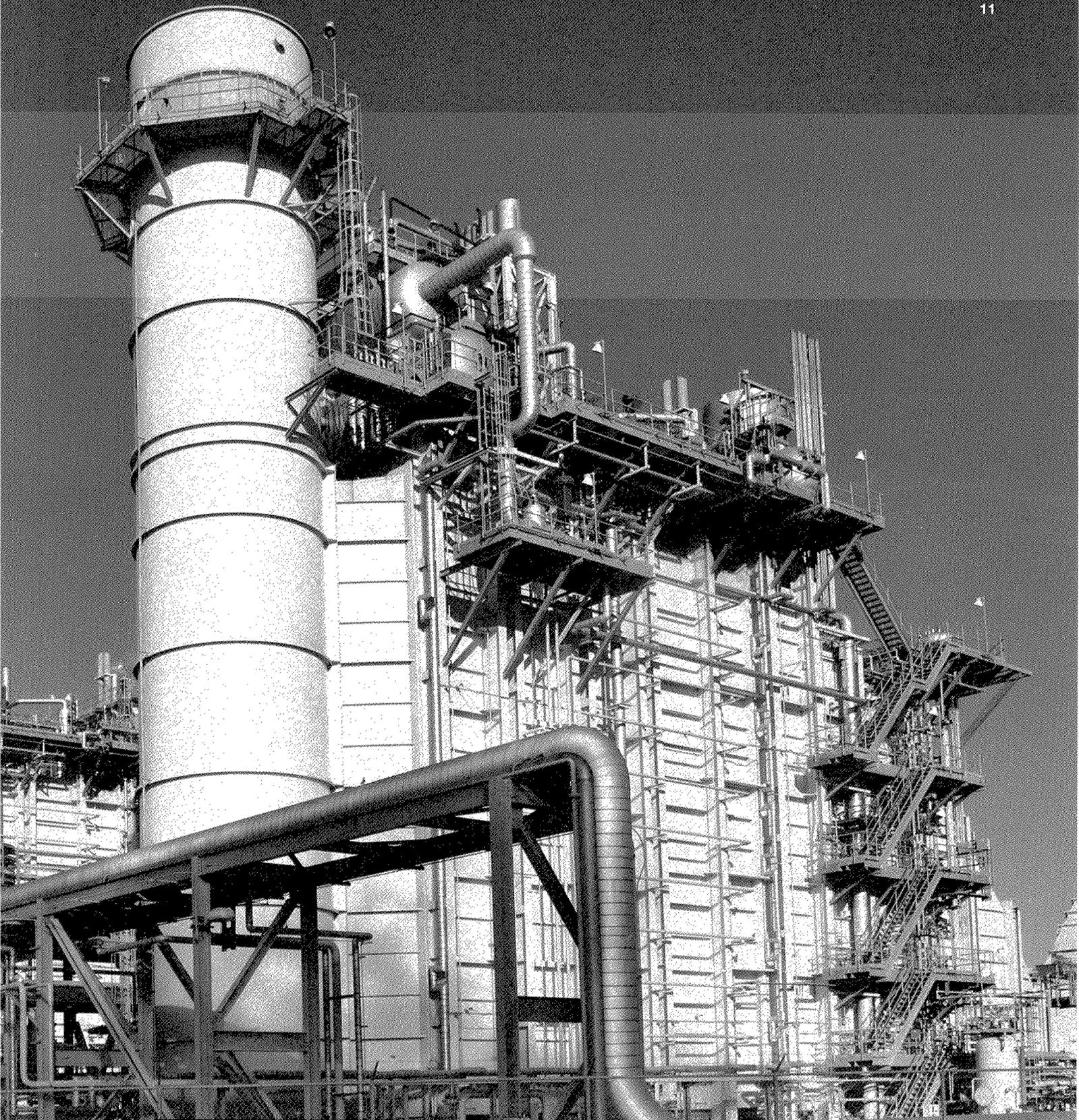
*At our refinery in Beaumont, Texas, one cogeneration plant – our largest worldwide – can produce about 500 megawatts of electricity, which not only powers refining operations but also supplements the local power grid.*
