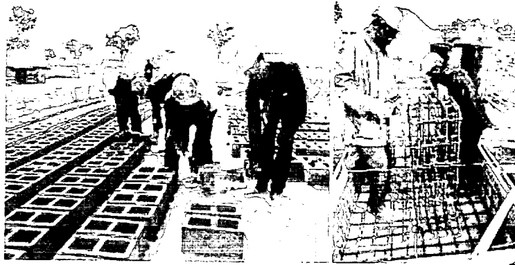
Moundou- and N'Djaména-based construction company Encobat has a contract to help build warehouse and workshop facilities at Komé Base Camp. Workers assemble rebar reinforcing steel (right) and make building blocks (left).
