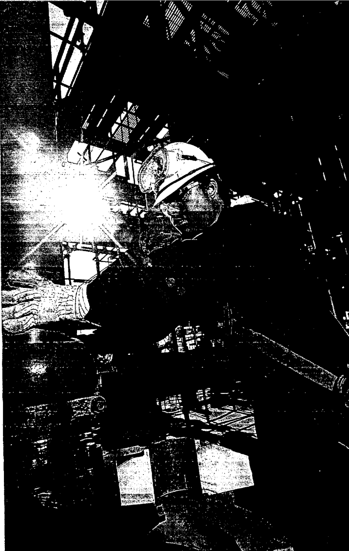
A worker prepares a cutting tool that removes petroleum coke from drums at the new Cerro Negro Upgrader Complex.
