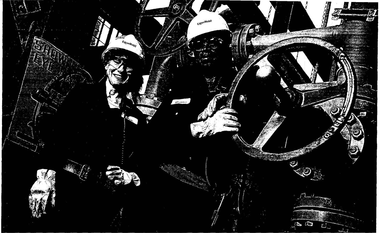
Installation of 67 pieces of new equipment and modifications to 50 others allow Lisa Muscarello and Forest Waters, operators at the Chalmette refinery, to help convert heavy crude.
