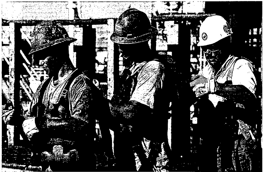
Crew members of ENSCO Rig 99, under contract to ExxonMobil, help each other secure harnesses and vests prior to being lifted in work baskets. These preparations are vital to safely carrying out the rig-maintenance activity shown below. "Nobody Gets Hurt" is about workers watching out for one another.
