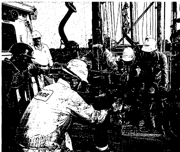
Development drilling is on track to reach a goal of more than two wells a week after the fall rainy season.
