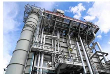
→ ExxonMobil has interests in more than 100 cogeneration facilities around the world, with the latest unit recently completed at Imperial's Strathcona refinery in Alberta, Canada.
