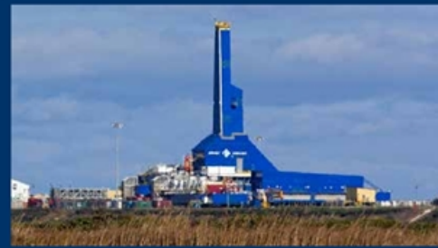
→ The Yastreb drilling rig, Sakhalin Island, Russia.
