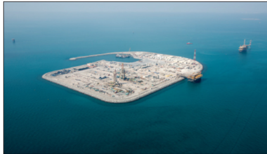
Drilling was initiated in 2014 from the artificial islands at Upper Zakum, United Arab Emirates, with plans to expand production to 750 thousand barrels per day.
