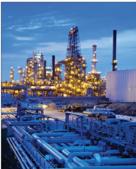
ExxonMobil is an industry leader in feedstock flexibility and challenged crude processing. For example, our Joliet Refinery is able to process significant volumes of lower cost, heavy Canadian crude.
