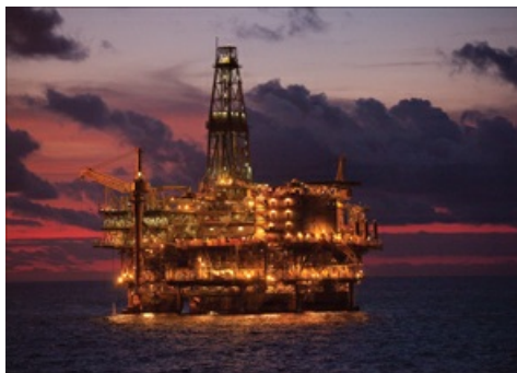
Angola Block 15 facilities, including the asset at Kizomba B, continue to operate with very high reliability.
