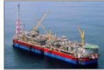
Deepwater Kizomba Satellites
