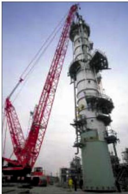
*Installation of the naphtha splitter fractionation tower at the Joliet, Illinois, refinery for production of low-sulfur motor fuel.*
