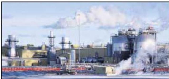
*The Cold Lake Mahkeses facility, which started up in 2002, includes a cogeneration facility. Heat recovery steam generators make steam to inject in the reservoir for improved oil recovery.*
