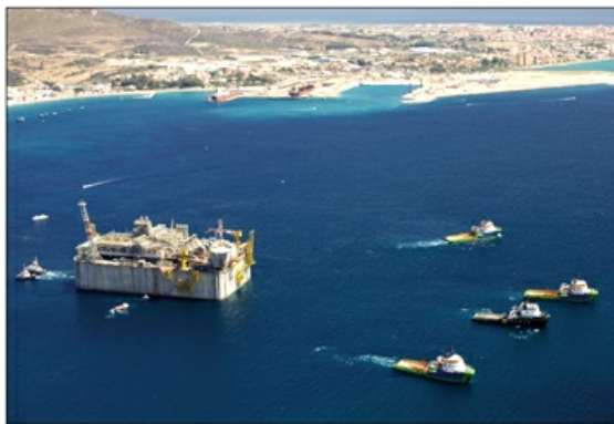
The Adriatic LNG terminal was towed from its construction site in Algeciras, Spain, to its final destination offshore Porto Levante, Italy. Commissioning activities are under way for start-up in 2009.
