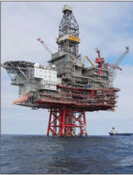
The ExxonMobil-operated Ringhorne platform is 110 miles offshore Norway in 410 feet of water.
