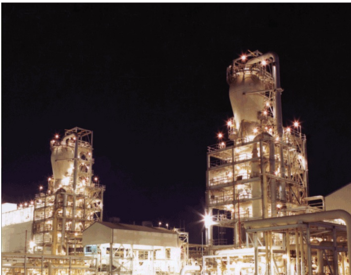
ExxonMobil's world-scale petrochemical facilities around the world enabled record earnings performance in 2006. The Kemya facility shown here is one of two successful joint petrochemical ventures in the Kingdom of Saudi Arabia with Saudi Basic Industries Corporation.
