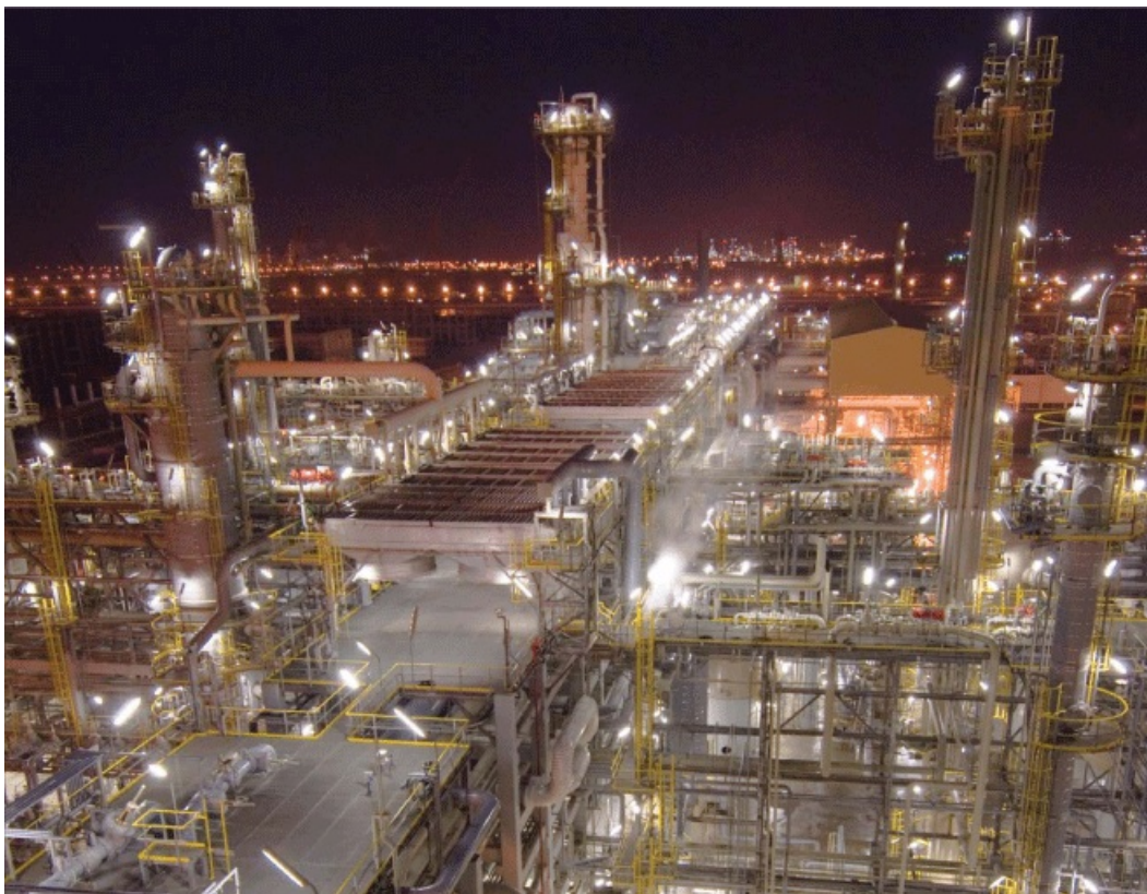
ExxonMobil and Qatar Petroleum began early production of LNG from Ras Laffan Liquefied Natural Gas Company II Train 5, 29 months after award of major construction contracts. The project was completed in early 2007 with the start-up of the offshore production facilities.
