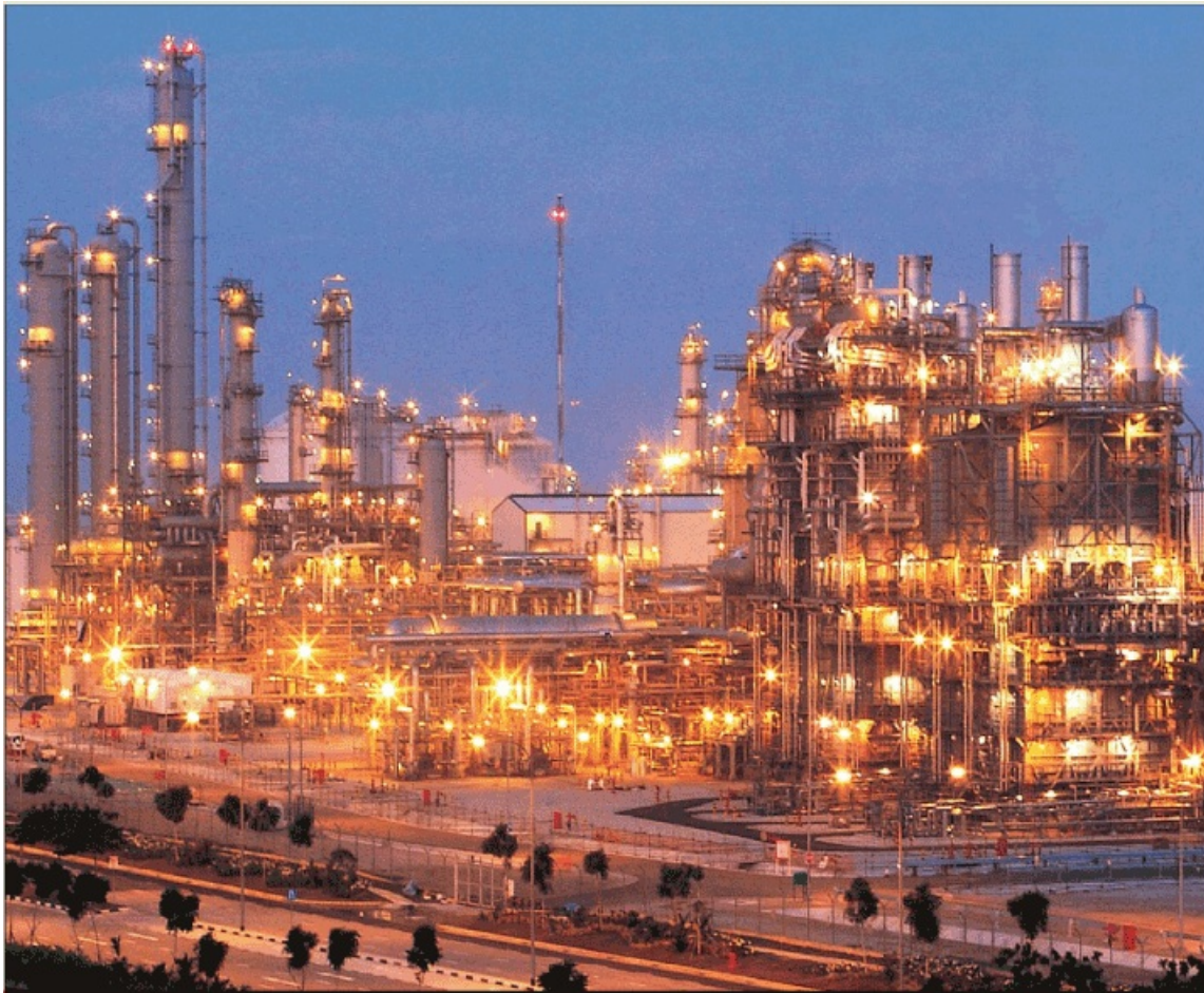
ExxonMobil's Singapore refinery is one of the largest in the world and is well-positioned to take advantage of the strong demand growth forecast in many countries in the Asia Pacific region.
