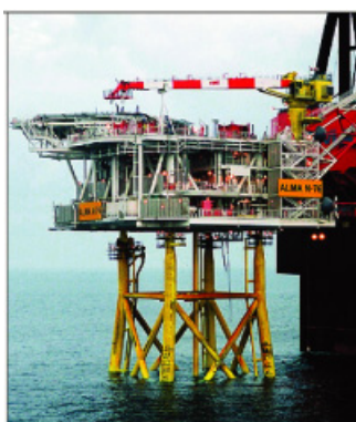
Installation of the Alma platform, part of the second phase of Sable Offshore Energy Project gas developments. This design will also be used for South Venture, scheduled to start up in 2005.
