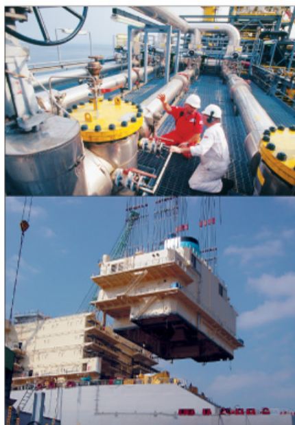
(Top) One of the ways the company leverages the breadth of our portfolio is the concept of "designing one and building many." The Zafiro Southern Area expansion was the second of the three deployments so far of the Early Production System (EPS).
