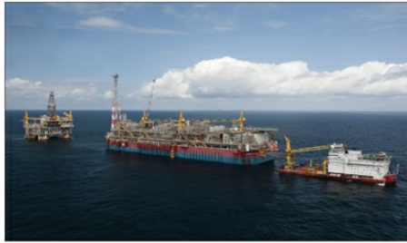
The Kizomba Satellites project in Angola is expected to start production in 2012.
