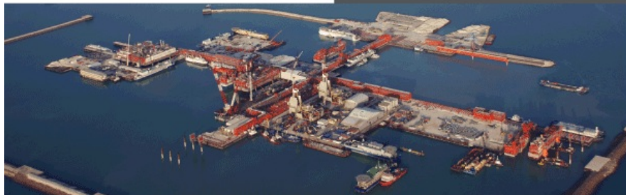
The Kashagan Phase 1 project uses artificial islands in the Caspian Sea to support drilling and production operations.
