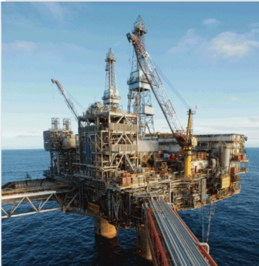
A new drilling program started at the North Sea Beryl field in 2009 that will develop additional reserves and extend field life.
