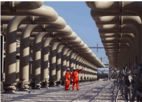
In 2009, ExxonMobil and our joint venture partner, Qatar Petroleum, started up three 7.8-million-tonnes-per-year LNG trains, the largest in service anywhere in the world.
