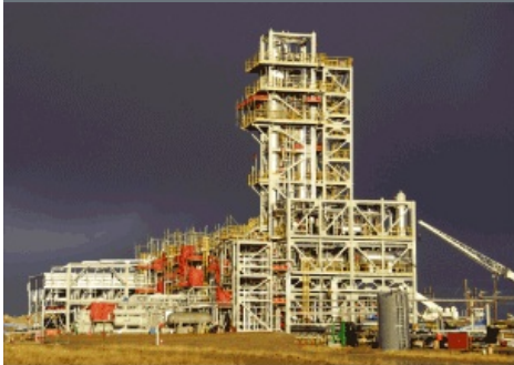
ExxonMobil's proprietary CFZ technology can remove CO 2 and H 2 S from natural gas in a single step, significantly lowering development costs for natural gas resources containing these impurities. Field testing will begin in 2010.
