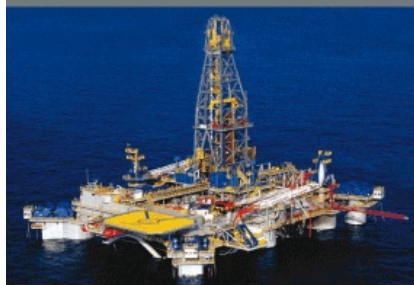
ExxonMobil began exploration drilling offshore Libya in 2009 using the Homer Ferrington semisubmersible rig.
