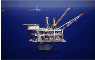
Stationed in over 4800 feet of water, the Hoover platform produces oil and gas from the Hoover field and several subsea tiebacks. In the background, the Ocean Valiant rig conducts development drilling at the Rockefeller discovery.
