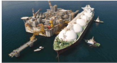
The Adriatic LNG Terminal is the world's first fixed offshore regasification facility and can supply about 10 percent of Italy's gas market needs. It received its first cargo in 2009.
